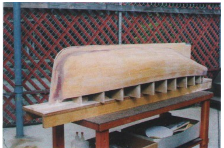
Building the hull of the Frances C
