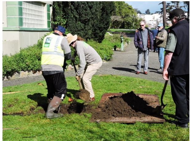
Park staff prepared the site.
